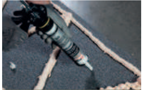
Tussenin dotten Recta Fix 'Alles + Alles' of Rectavit G60 'High Tack'/ G70 'Heavy Duty'
